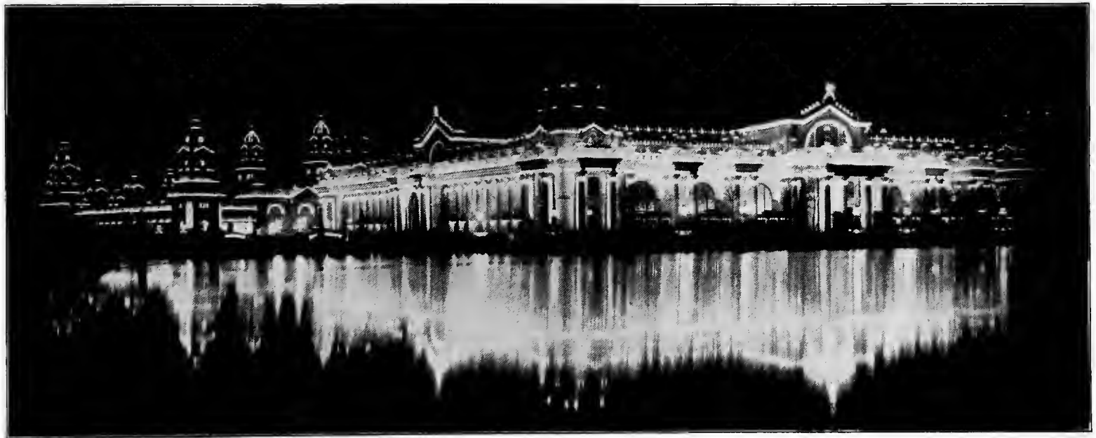
PALACES OF MACHINERY AND ELECTRICITY AT NIGHT.
